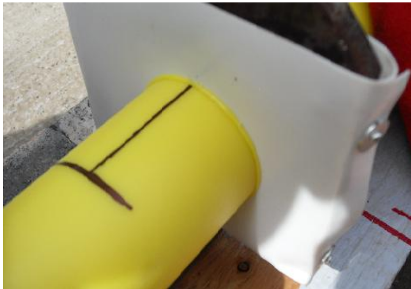
Figure 21. Formation of molten plastic bead around perimeter of pipe
