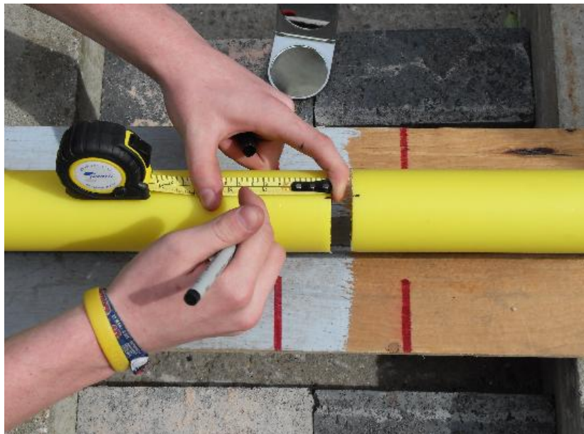
Figure 20. Alignment and marking of pipe ends
