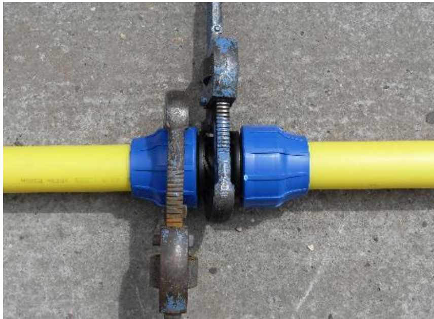
Figure 22. Tightening of compression nut using pairs of Stilsons
